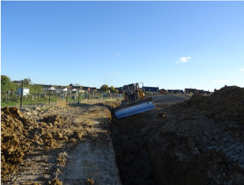
Forming the swale/ ditch on the eastern boundary in October 2017
