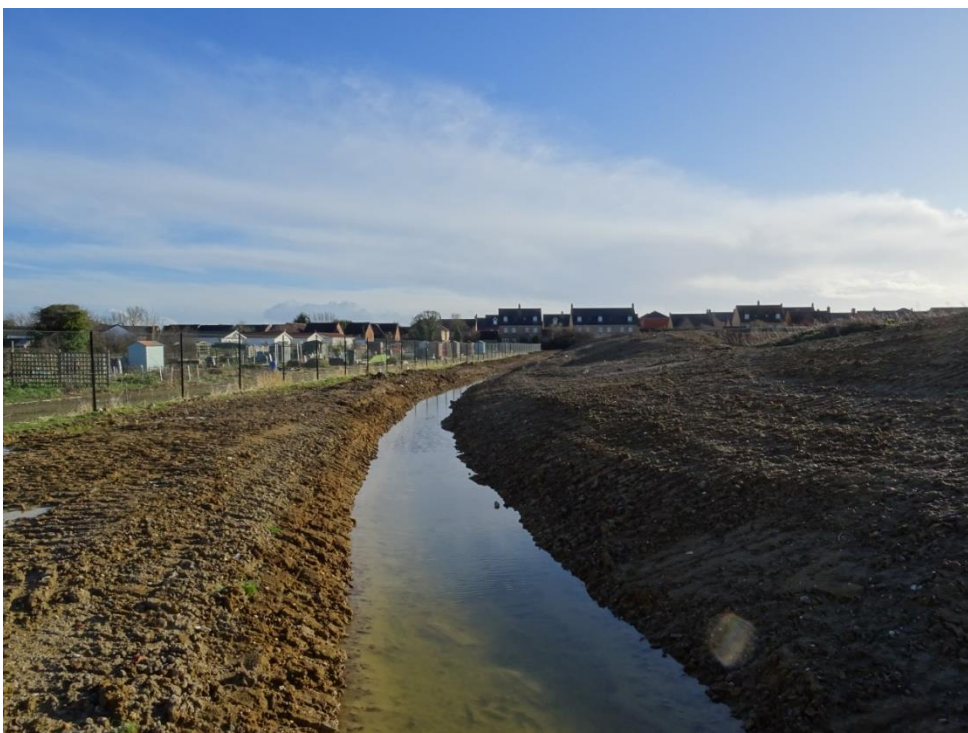
The allotments on the eastern boundary had flooding problems during the winter months but the forming of the swale/ditch has alleviated the problems for the allotment holders.
