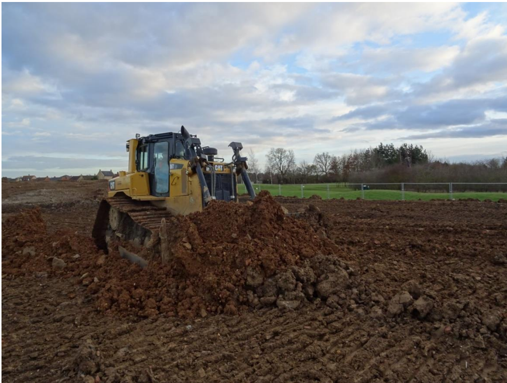
Commencement of filling operations for 14th tees
